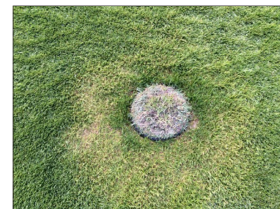
Fig 60. Dangerous irrigation sprinkler within the field of play.
