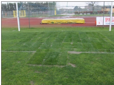
Fig 38. Poor surface levels in a re-turfed goalmouth.
