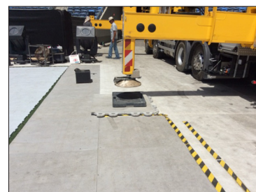
Fig. 87. Heavy-duty panelling to support large vehicles and cranes.
