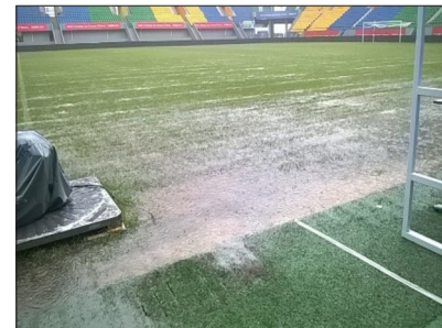
Fig 44. Heavy rainfall on a pitch with poor surface drainage – such conditions can lead to matches being abandoned.
