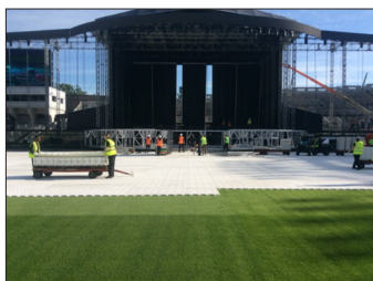
Fig. 89. Panelling is brought onto the pitch in untied loads, by small buggies that go back and forth hundreds of times.
