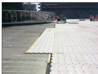
Fig. 90. Overlaying light-duty turf protection panels to provide a smooth transition onto the heavy-duty aluminium trackway panels on the left of the photo.
