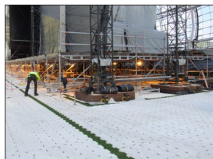
Fig. 93. Artificial lighting used to help grass survive under a stage.
