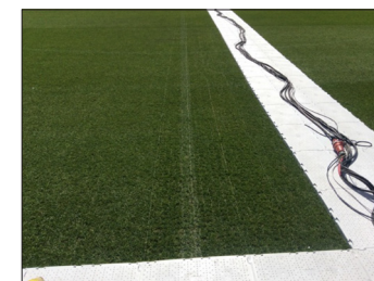
Fig. 98. Cables placed along protective panels to prevent potentially significant turf burn, while also creating a pathway for foot traffic across the pitch.
