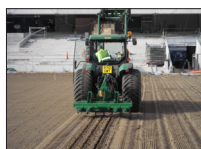
Fig. 7. Installing undersoil heating pipes through the profile
