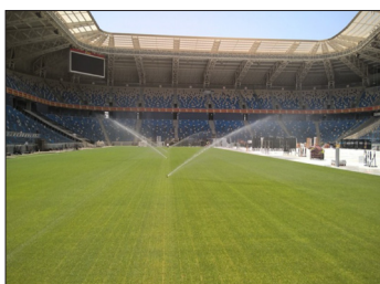
Fig. 105. An irrigation system with individual head control, used to water parts of the pitch while the turf protection system is still being removed.
