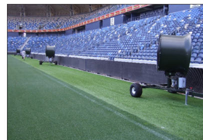
Fig. 11. Examples of pitch side ventilation and cooling fans used to manage turf health
