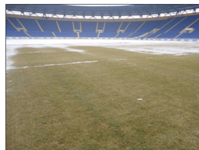
Fig 45. Poorly performing under-soil heating system failing to keep the surface uniformly free of frost and snow.
